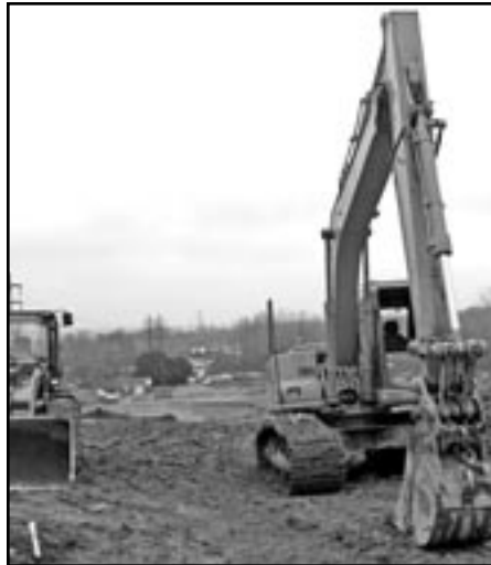
Construction of Hoover Lofts is just beginning. The project will be complete in August 2007.
